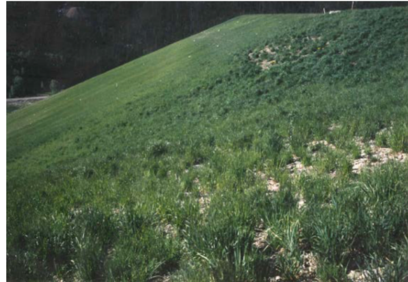
Mayflower Tailings pond 2, 1995 (after) – SGC moved the impoundment toe back from Boulder Creek and the highway to minimize the potential for erosion and migration. SGC flattened the side slopes to increase stability and potential for re-vegetation, regraded to promote drainage, capped with subsoil, and seeded.
