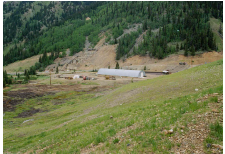
American Tunnel, 1998, (after) – SGC removed 80,000 tons of mostly historic mine waste and tails.
