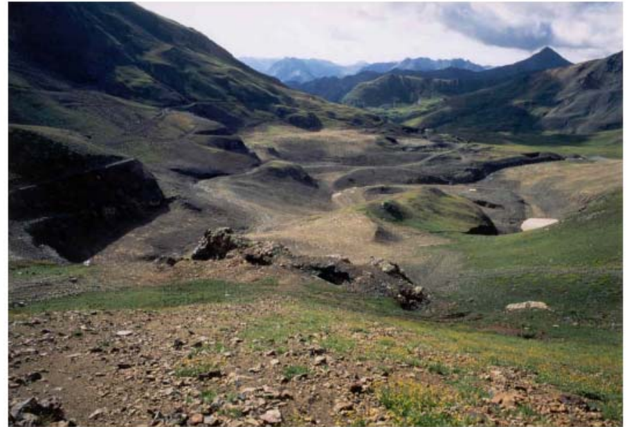
Sunnyside Basin, 1996 (after) – SGC placed 240,000 cubic yards of clean fill to cover the Lake Emma subsidence area and to create positive drainage, contoured the area, and seeded.
