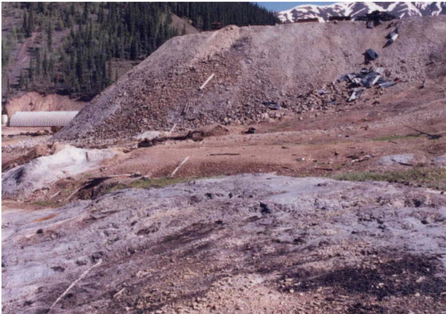
American Tunnel, 1995 (before)
