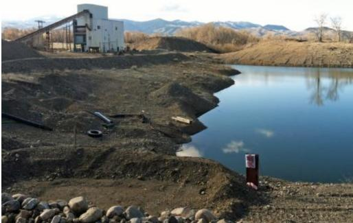
ALDER GULCH MINE SITE – West fresh water supply pond (previous dredge pond) next to active mining area converted to ore staging with wet plant in background
