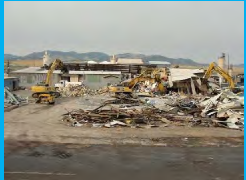
COAL MILL AND SODIUM BUILDING DEMOLITION
