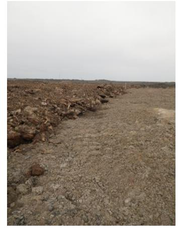
**Reclamation in progress** Forest floor – mineral mix being spread on top of overburden
