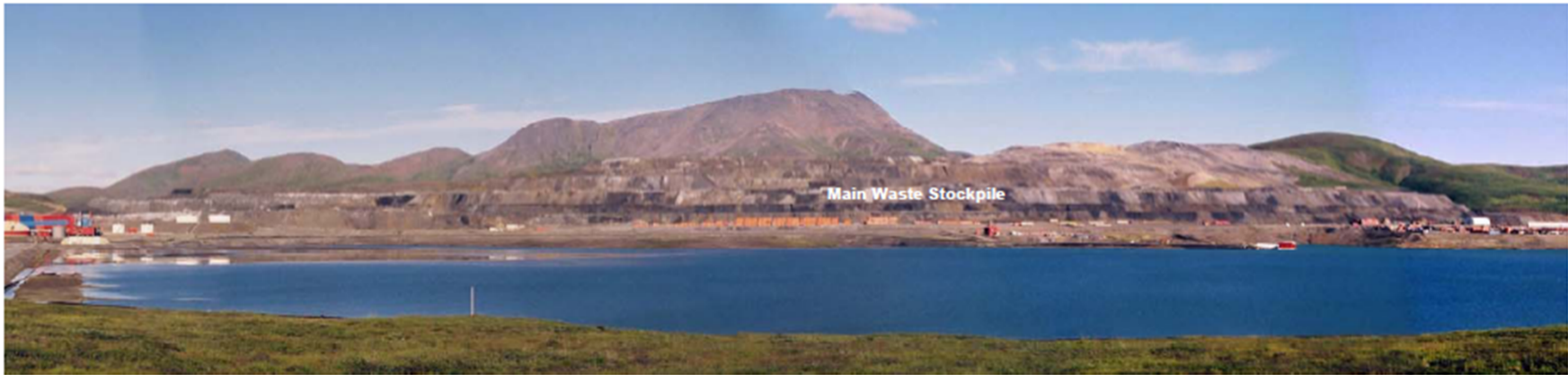
Current View of Main Waste Stockpile
