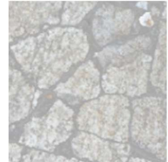
Impermeable Seal Created
